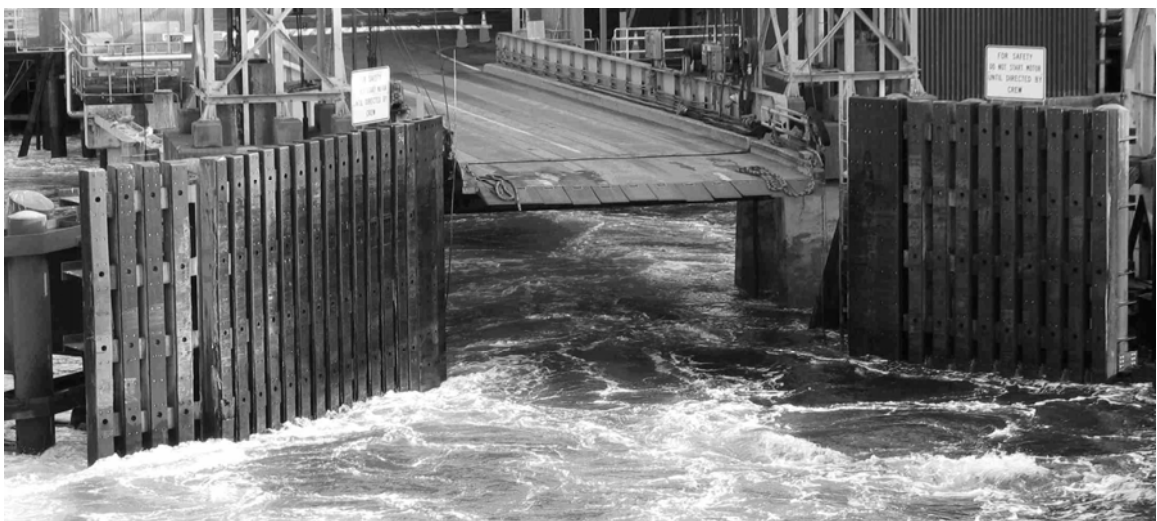
Figure 1.1 Ferry Landing Wingwall Structure.
